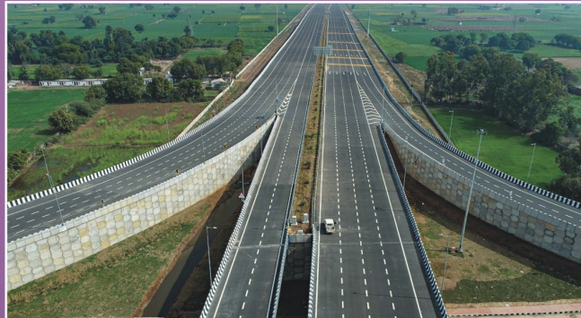
New Six lane Express Way
