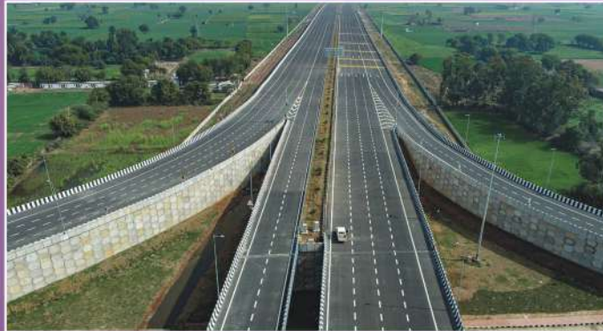
New Six lane Express Way
